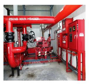
Fire hydrant installation consists of a system of pipe work connected directly to the water supply main to provide water to each and every hydrant outlet and is intended to provide water for the firemen to fight a fire. The Fire Hydrant Line is always kept pressurized with water. Afirefighter connects a fire hose to the fire hydrant and releases a valve to get water from the water main.
