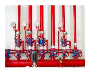
An automatic sprinkler system is intended to detect, control and extinguish a fire, and warn the occupants of occurrence of fire. The installation comprises fire pumps, water storage tanks, control valve sets, sprinkler heads, flow switches, pressure switches, pipe work and valves. The system operates automatically without human intervention
